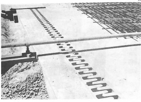
On the Sweetwater bridges they have nearly completed the steel expansion joiners, which look like serpentine designs. The fingers can expand into one another when it is hot, retract when the concrete cools, so it will not buckle or break. They have a movement length of about 3 inches. At right is some reinforcing steel used in completing the highway portion. The two bridges are finished.
